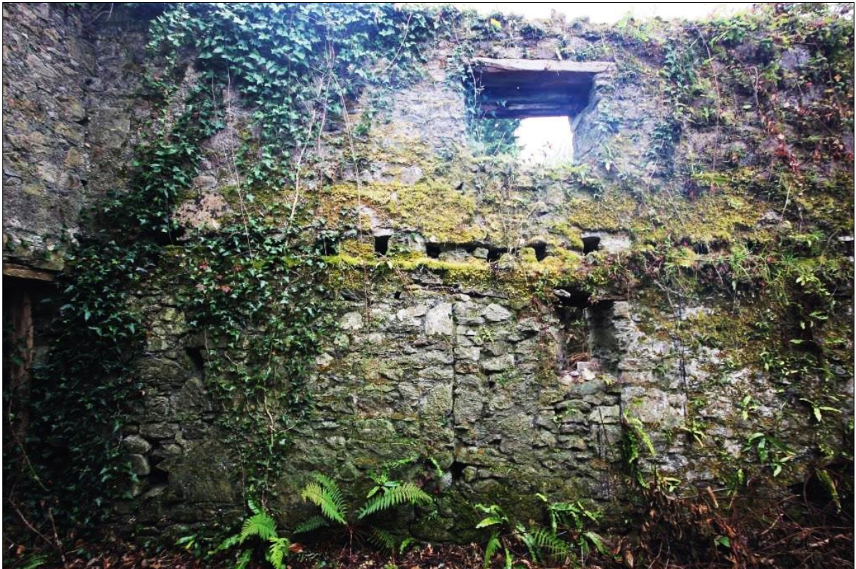
Plate 32: Putlog holes for floor joists and blocked up doorway
