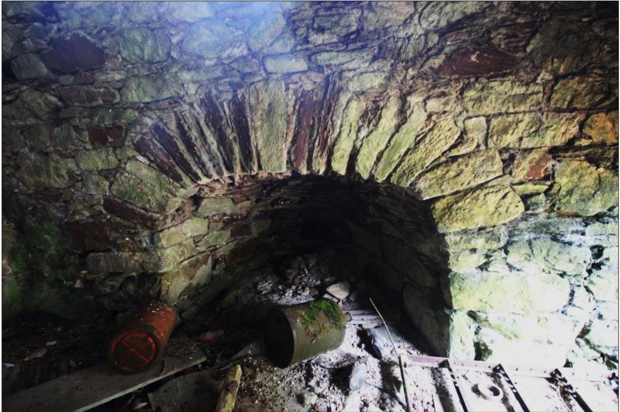
Plate 13: Lime kiln drawhole
